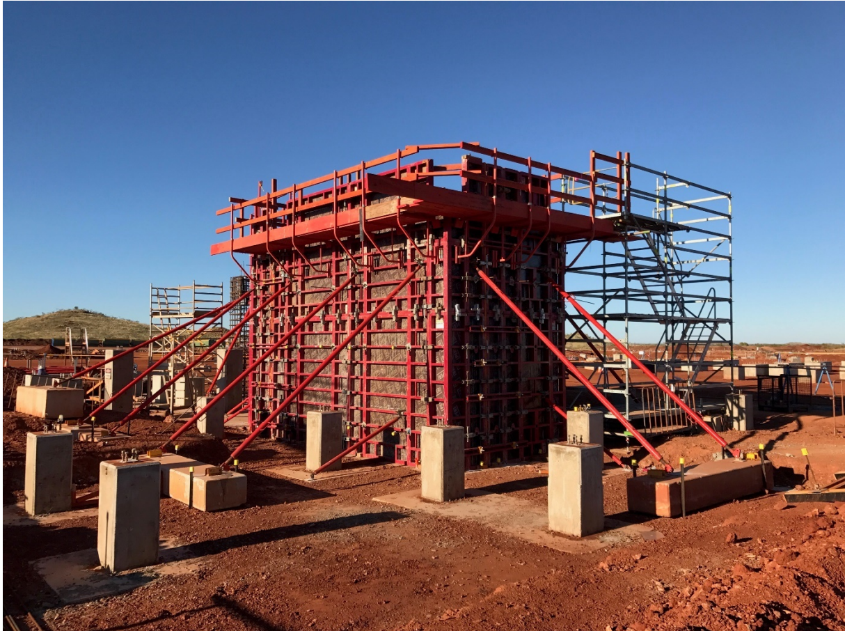
Figure 1 – Concrete Pour on the Main Part of the Ball Mill Foundation
