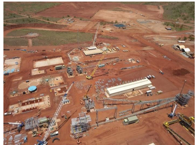
Photo 2 Construction in Progress from the western side of the Plant
