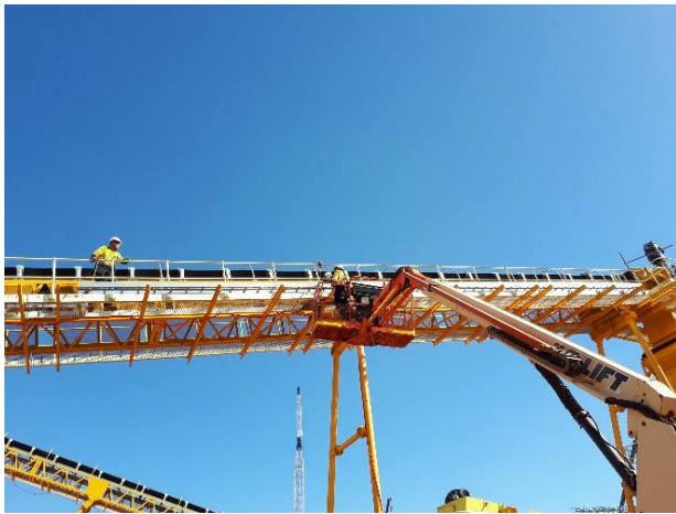
Photo 4 First Cable Tray installed on site
