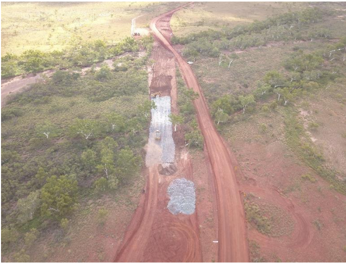
Photo 7. Wodgina Road Works
