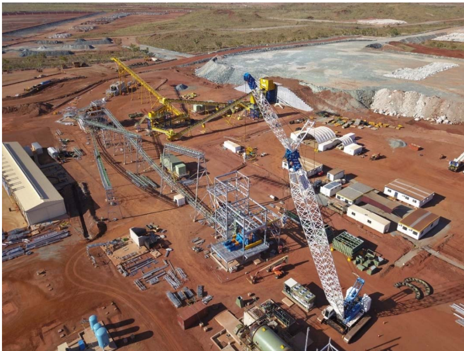
Mine site works nearing completion at the Altura Lithium Project
