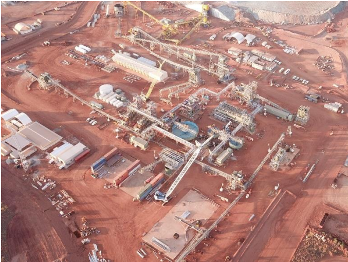
Photo 3 Process Plant Overview
