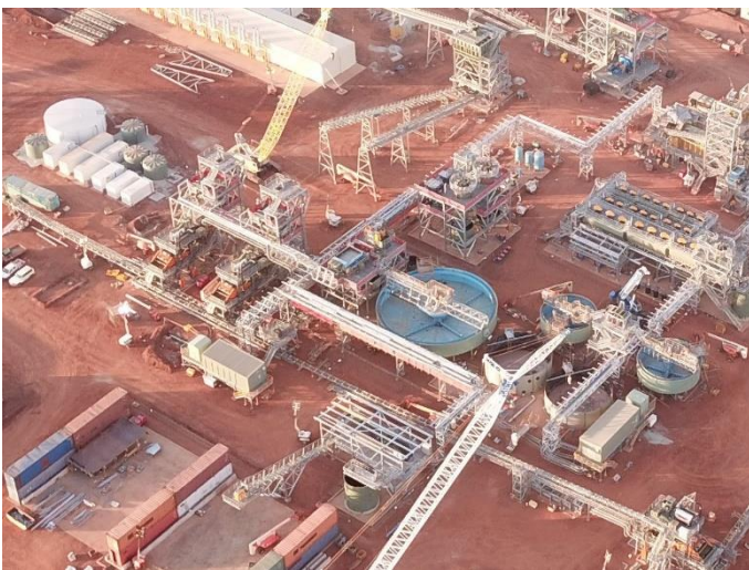
Photo 4 Completion of conveyors – erection of pipe racks
