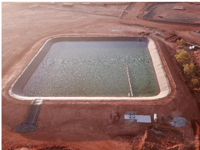
Photo 8 Raw Water Dam
