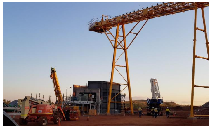
Photo 2 Installation of 2nd tier of Crushed Ore Bin
