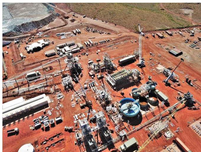
Photo 2 Mill from east
