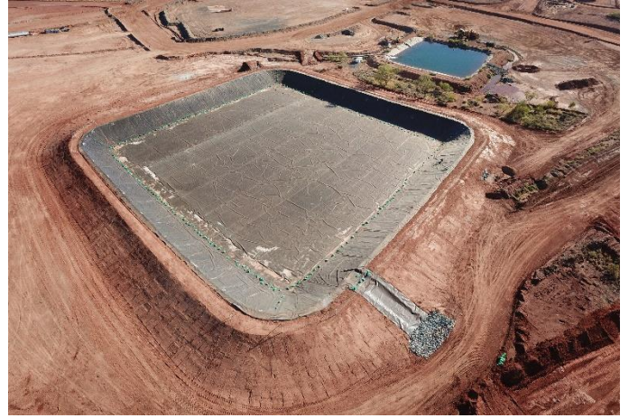
Photo 10 Raw Water Dam
