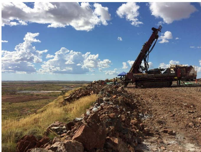
Photo 1 Drilling Activities at Southern Ridge
