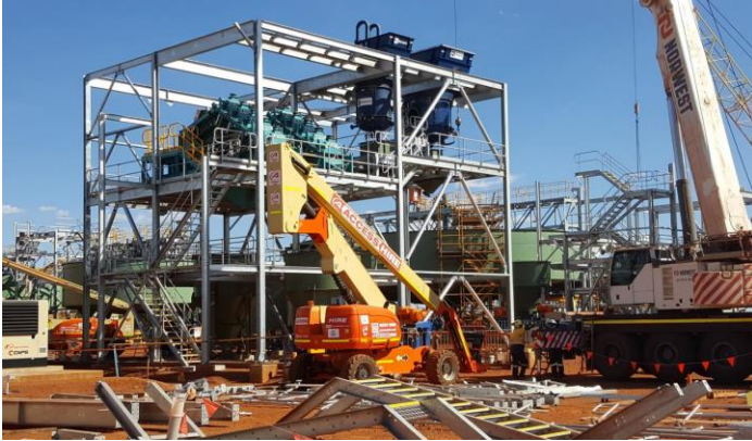
Photo 3 Installation of High Frequency Screens
