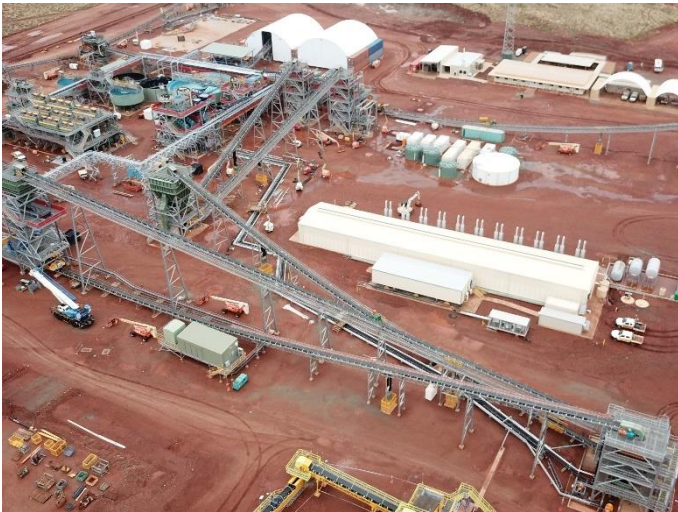
Photo 4 Conveyor sections installed
