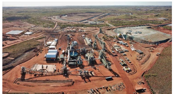
Photo 3 Processing Plant Overview
