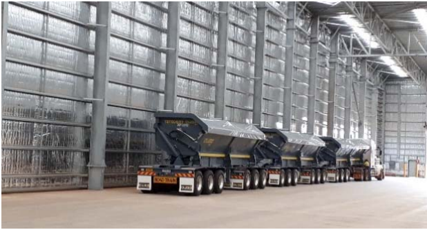
Photo 4 Inside Altura/QUBE Shed
