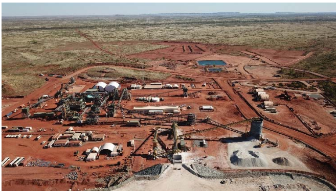
Photo 1 & Below Crushing – Building the Crushed Ore Overflow Stockpile
