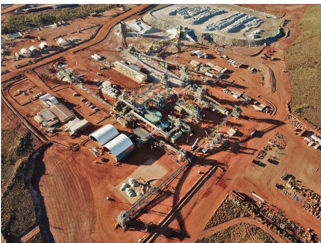
Photo 5 Processing Plant Site Overview
