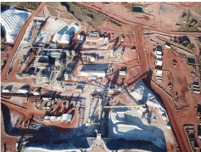
Photo 1. Altura Lithium Process Plant
